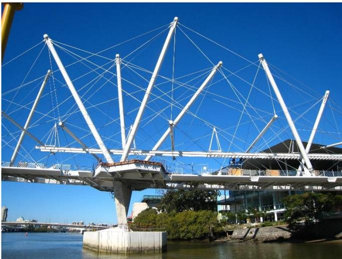
**Figure 5 Kurilpa tensegrity bridge in Brisbane Australia.** Image from Wikimedia Commons [19].
