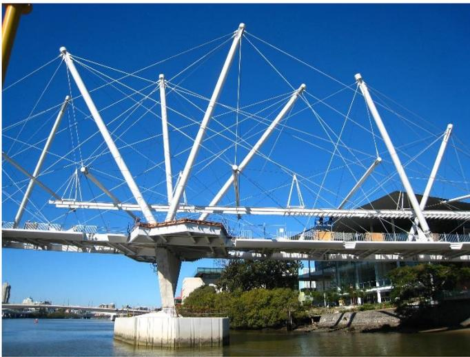
**Figure 5 Kurilpa tensegrity bridge in Brisbane Australia.** Image from Wikimedia Commons [19].
